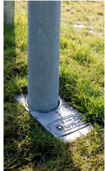
Lockable base and sleeve into which the post is inserted.
